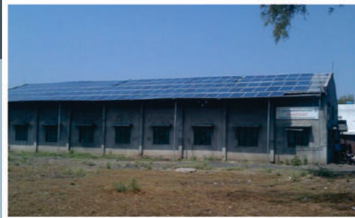
50KWP Solar Power Plant at Engg. College
